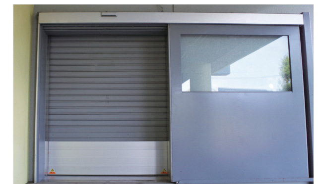
Shutter with water stop plate
