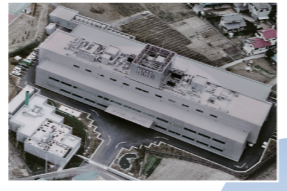
November 1984 Completed construction of the laboratory building at BML General Laboratory
