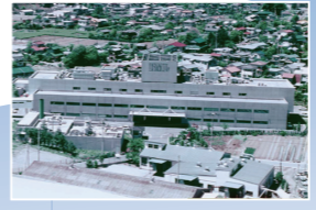
June 1987 Completed construction of the office center at BML General Laboratory
